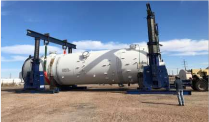
700-ton LIFT-N-LOCK® Gantry System
